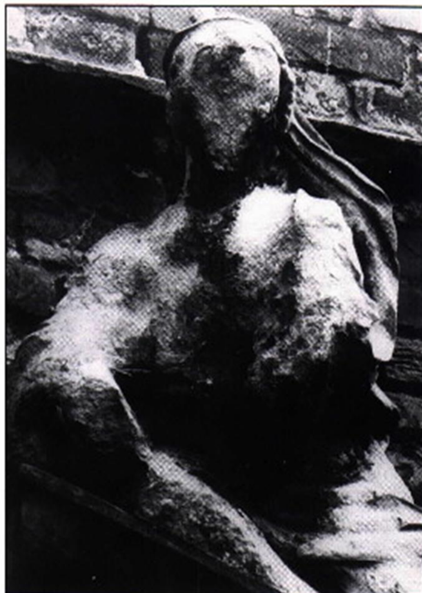
Fig. 11. A sandstone figure on an early eighteenth-century building in Germany shows the effects of twentieth century air pollution. The photograph on the left dates from 1908, the one on the right from 1969. Calcium-containing stones such as limestone and sandstone are particularly vulnerable, but other materials, including brick, concrete, glass, and metal, are also affected.
