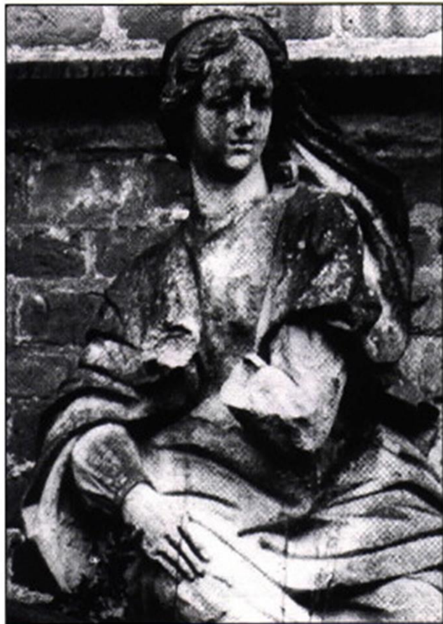
Fig. 11. A sandstone figure on an early eighteenth-century building in Germany shows the effects of twentieth century air pollution. The photograph on the left dates from 1908, the one on the right from 1969. Calcium-containing stones such as limestone and sandstone are particularly vulnerable, but other materials, including brick, concrete, glass, and metal, are also affected.
